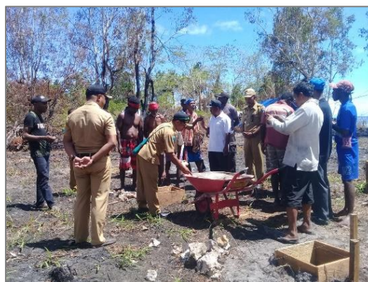
Placement of Patrol Post First Stone
